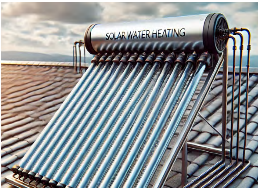
An example of solar thermal panel installation on a house rooftop
