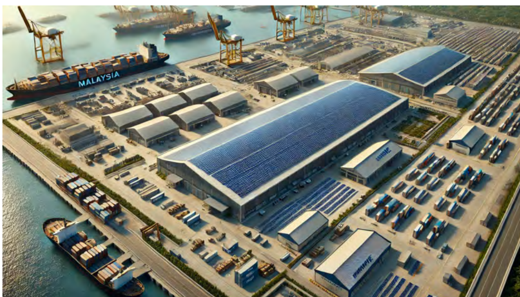
Figure 2: Installation of large-scale PV solar on the roof
