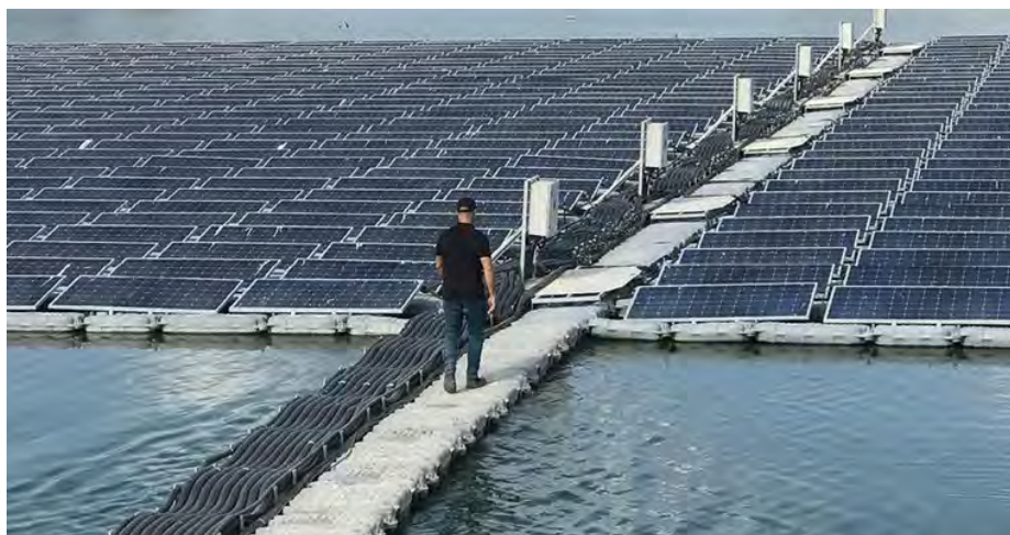
Figure 12 Floating walkways for floating solar farms
