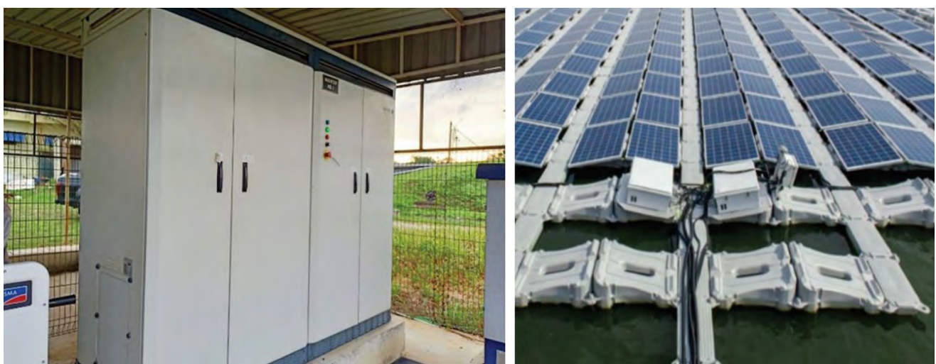
Figure 3 String inverter for solar farms on land and on water
