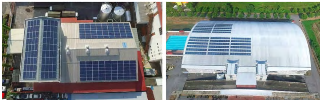
Figure 15 Example of PV installed following design and not exceeding the highest or edge of the building roof
